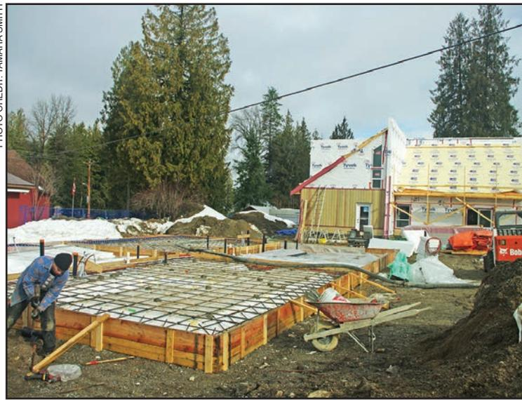
Installing wall supports before the pour for Unit 2 of Slokan City Suites.
